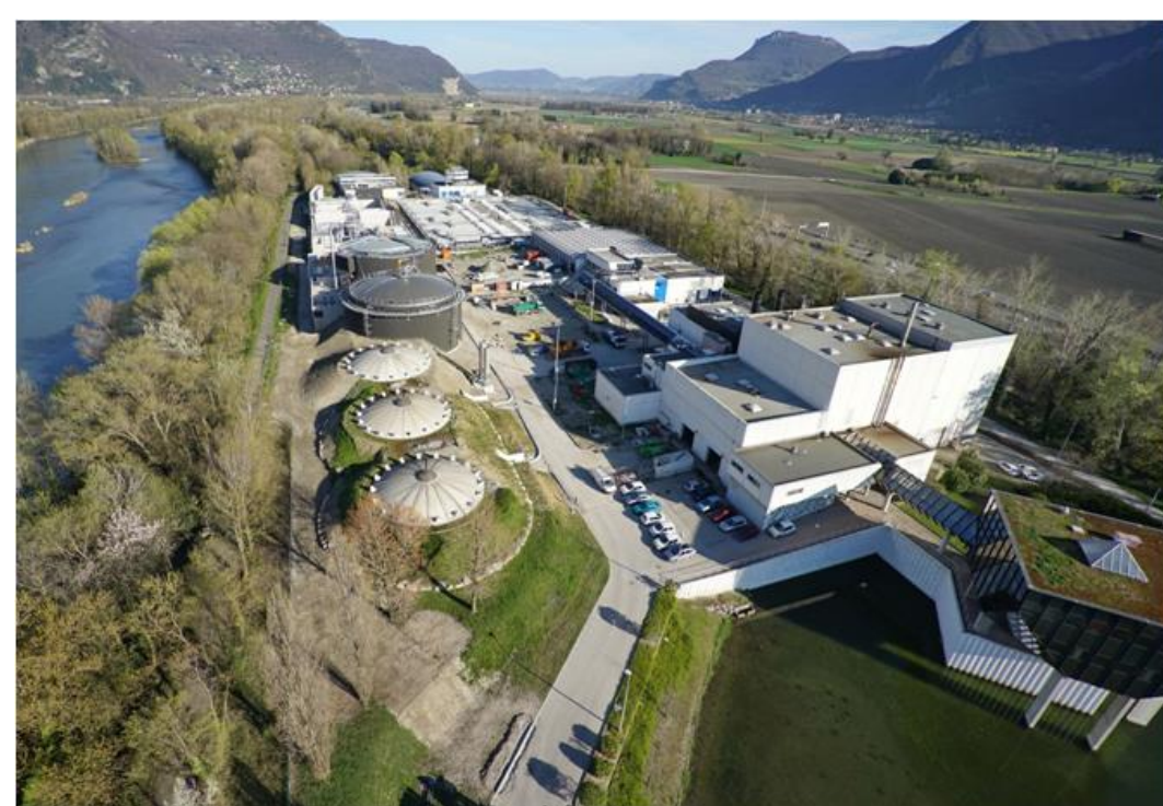
Grenoble metropolis wastewater treatment plant facility(AQUAPOLE)
